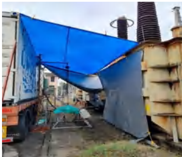
Figure 14: Sodium mixer area covered with tarpaulin sheets
