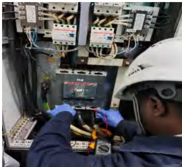
Figure 6: Power supply connections to control panel
