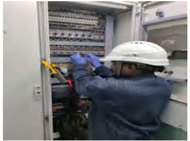
Figure 9: Checking the electrical connection for main control panel
