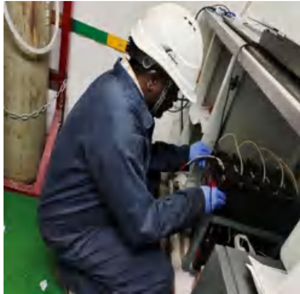
Figure 16: Battery replacement
