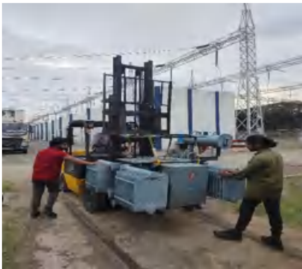
Figure 3 :Unloading of PCB accessories such as step down transformer, sodium dispersion drums etc.
